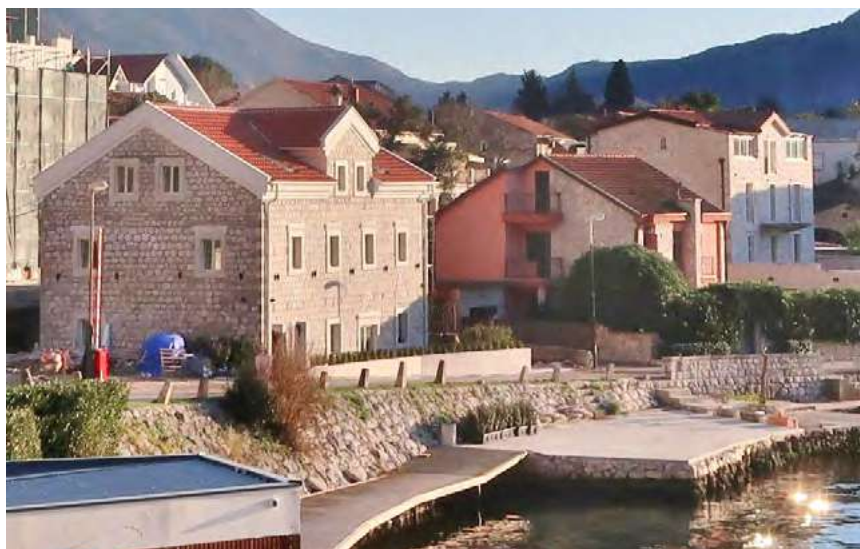
Fig. 11a, b and 12a, b: Kavalin area in Dobrota, and detail of traditional house (2018) and after restoration (2025). Parallel to the new constructions, there are also cases of inappropriate restoration works on traditional buildings. In this traditional house, original stone window frames - previously in good condition - were removed and replaced with profile dimensions and stone type that are not in accordance with the traditional ones. The authentic roof cornice was replaced by a new oversized and profiled cornice that is not at all characteristic of the traditional architecture of Bay of Kotor.
