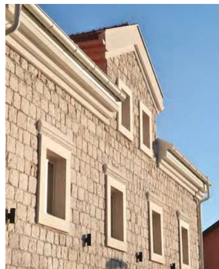
Fig. 11a, b and 12a, b: Kavalin area in Dobrota, and detail of traditional house (2018) and after restoration (2025). Parallel to the new constructions, there are also cases of inappropriate restoration works on traditional buildings. In this traditional house, original stone window frames - previously in good condition - were removed and replaced with profile dimensions and stone type that are not in accordance with the traditional ones. The authentic roof cornice was replaced by a new oversized and profiled cornice that is not at all characteristic of the traditional architecture of Bay of Kotor.
